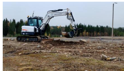
The Smart Excavator in 5G Private Network
