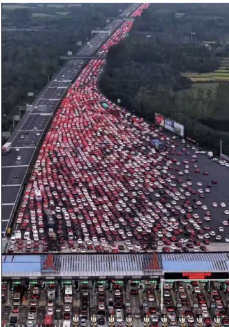
China's Wuzhuang toll station, 36 lanes stuck on 8 th October 2025
